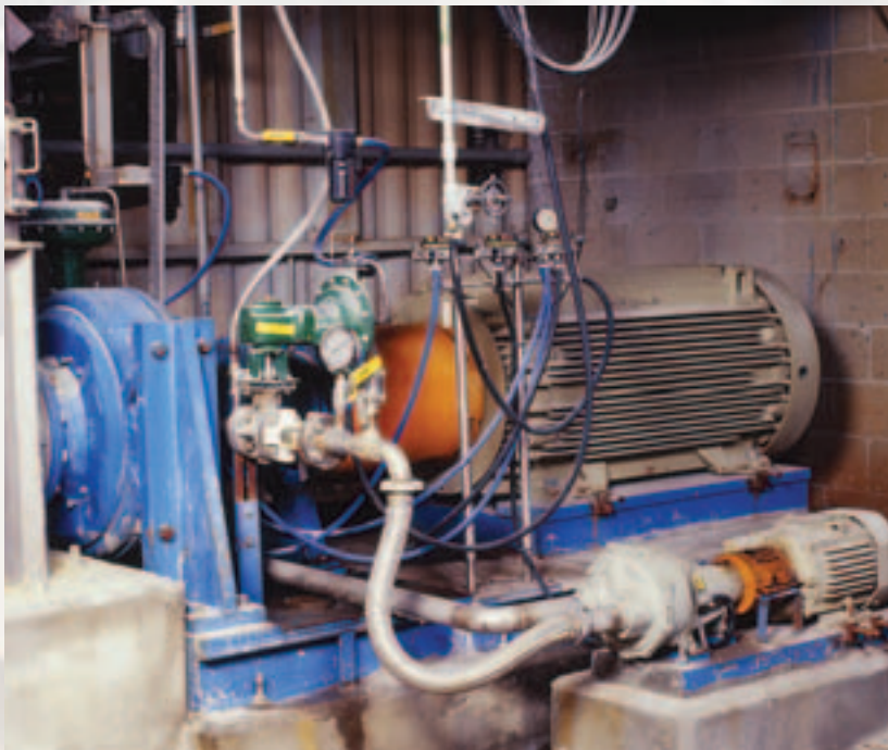
Bleached pulp from final wash stage being pumped to HD storage.
