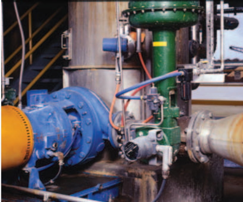
Caustic stage pumping from washer operating at 1200 TPD at 12% consistency. One of seven units in complete bleach line.
