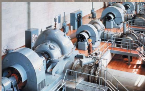
A-C split case pumps have many applications in the power generation market.
