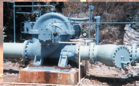
Split case pump in service at an electric utility plant in the Bahamas.
