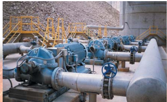
All 316 stainless steel 9100 series pumps on a solvent extraction application at a large copper mine.
