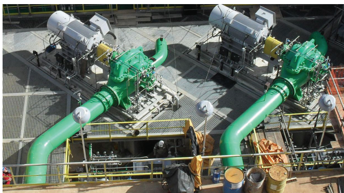
Brazil Refinery Cooling Tower Service
