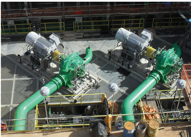
Refinery Cooling Tower Service (Brazil)
