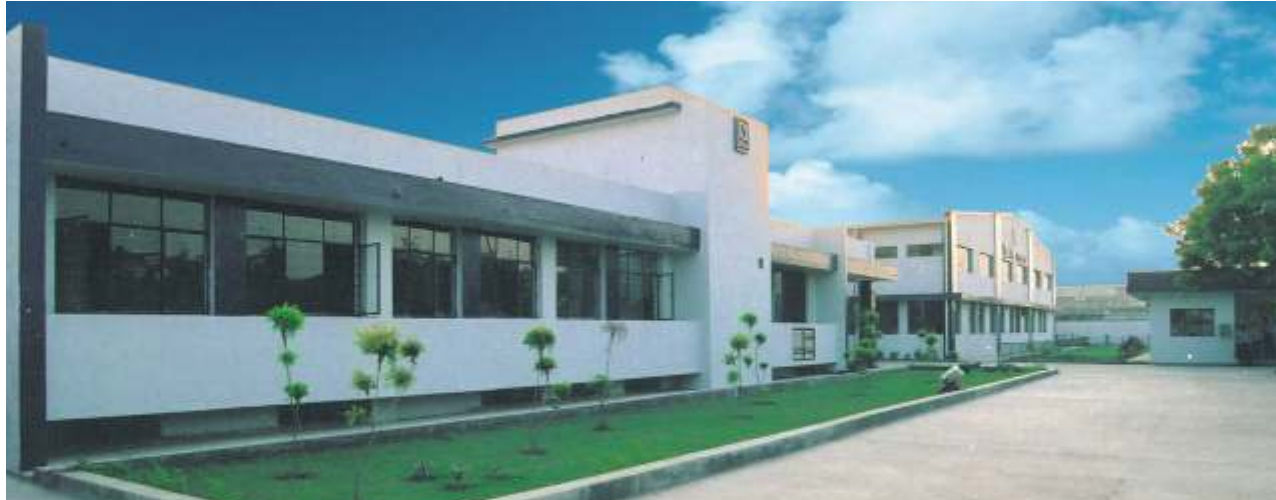
Roto's Manufacturing Plant
